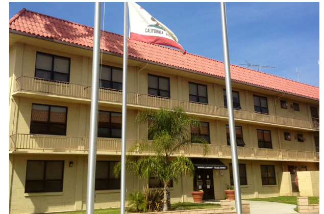
The Ben Clark Training Center Administration/Classroom Building is a repurposed facility originally built for March AFB.
