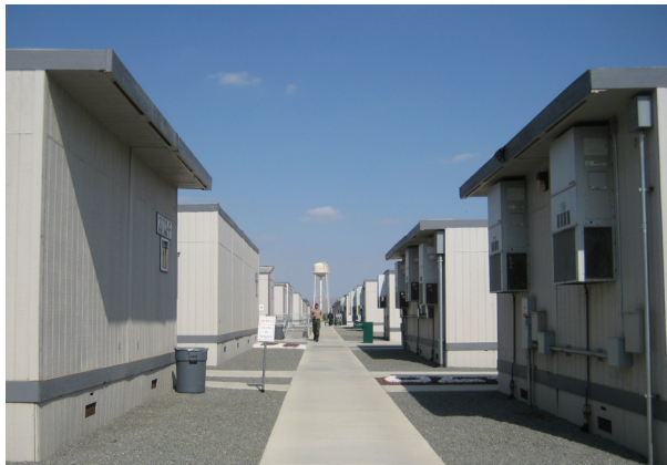
Law Enforcement temporary relocatable classrooms
