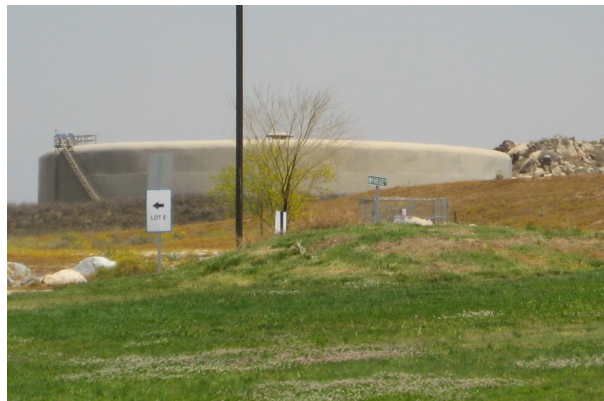
EMWD Water Tanks
