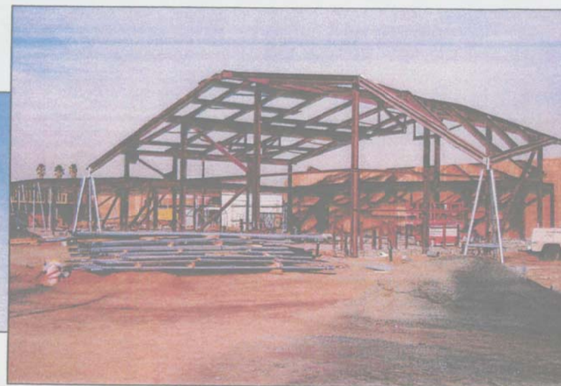
The Learning Center Construction Progress- Museum Building and Building L
