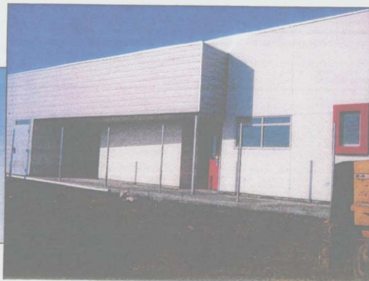
The Learning Center Construction Progress-Building F
