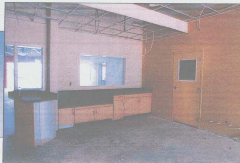
The Learning Center Construction Progress- Typical Interior Classroom Casework
