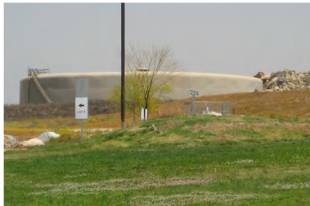
EMWD Water Tanks
