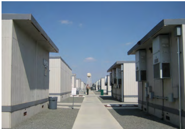
Law Enforcement temporary relocatable classrooms
