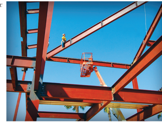
Norco Industrial Technology Complex
