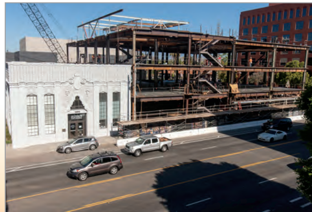
Centennial Plaza construction
