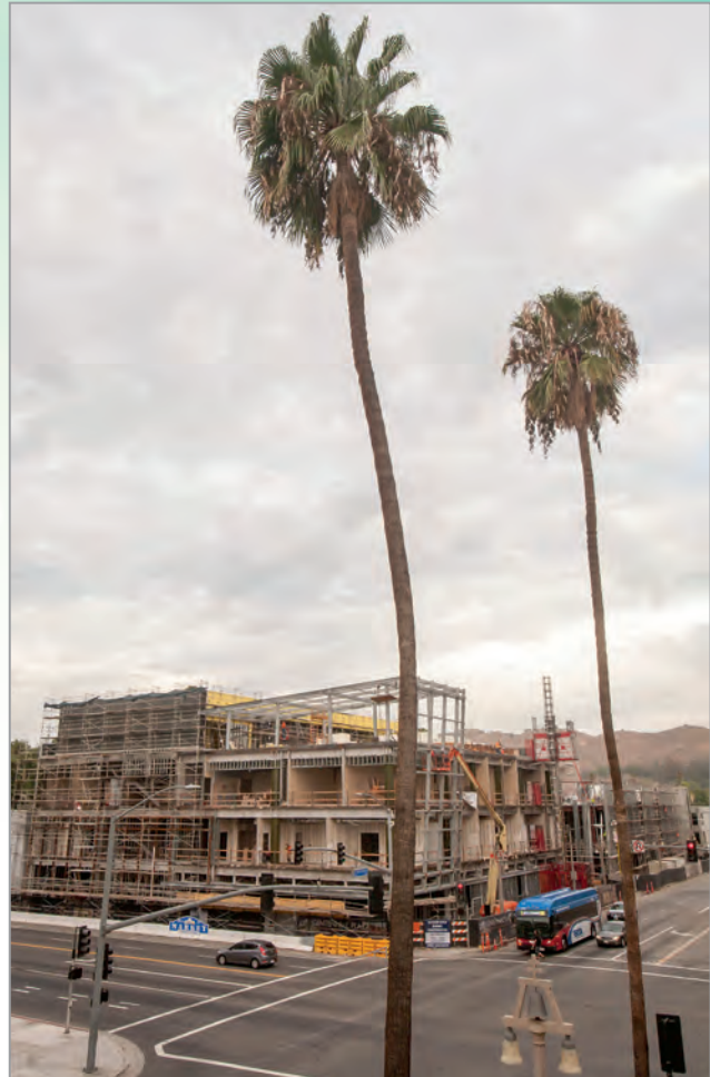
Centennial Plaza construction
